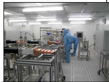
EU-XFEL : Preparation and power testing of 800 couplers
