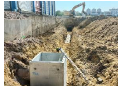
June 2023 : reorganization of site utilities
