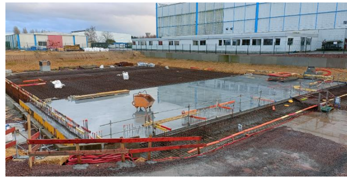
January 2024: Finishing of level -3 wall
