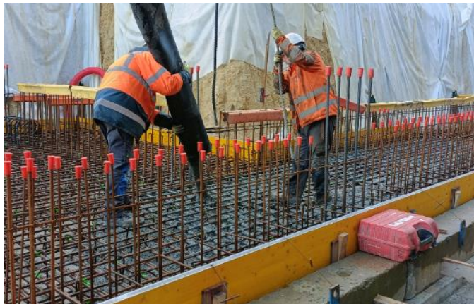
October 2023 : First concrete!
