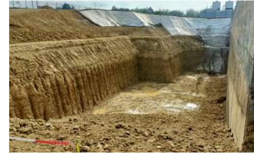
July 2023 : general earthworks
