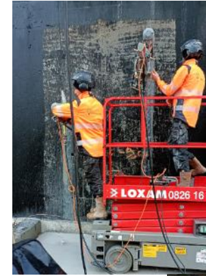
Drilling of existing walls, elevation of walls to level -3 and preparation of hall floor slab
