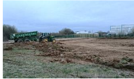
April 2023 : surface levelling
