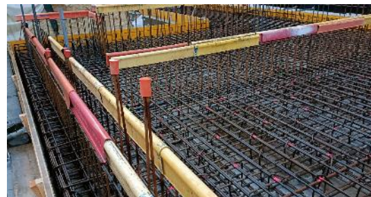
October 2023 : steel reinforcement level -3
