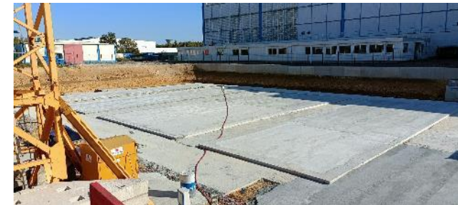
October 2023 : Surface preparation
