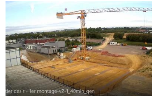
September 2023 : Site preparation
