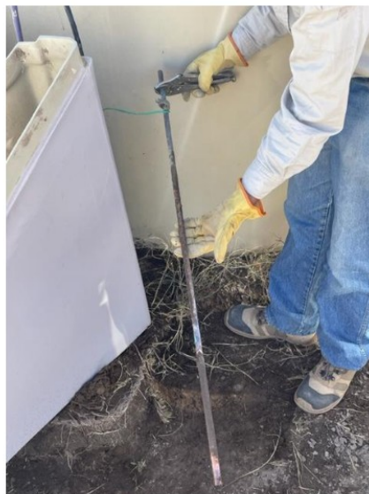
Figure 4 : Grounding rod in Saturno.
