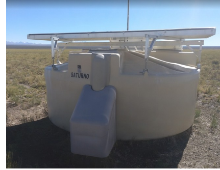
Saturno (1093) - SSD-cable - sPMT-cable - grounding rod
