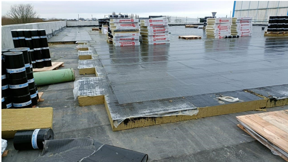
Thermal isolation of roof
