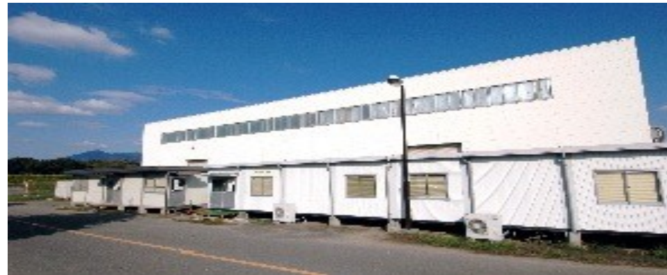
Figure 3: KEK ATF assembly hall building photo
