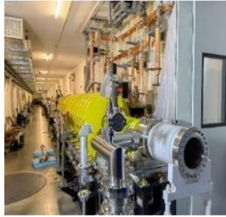
May 12, 2022 The Linac Vacuum-sealing in the tunnel completed
