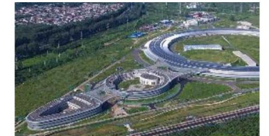
Nov. 3, 2023 Civil Construction for ancillary buildings completed
