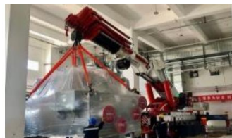
Apr. 13, 2021 Utility installation in NO.2 Hall commenced
