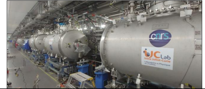
ESS : - preparation & testing of cavities, couplers and tuners - Integration of 14 cryomodules
