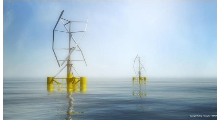
Floating vertical axis wind turbine VERTIWIND Project
