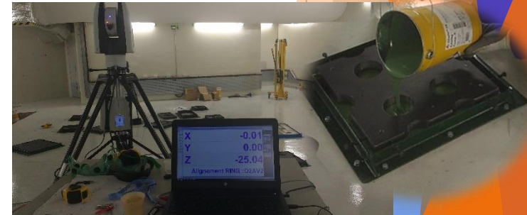
Bonding of the Steel plates on the bunker ground
