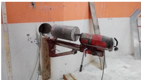
Drilling of the X Line penetration
