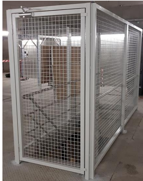
Access to basement area
