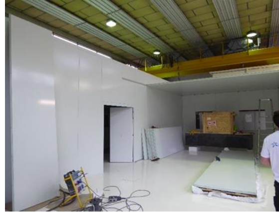
Construction of an ISO7 clean room
