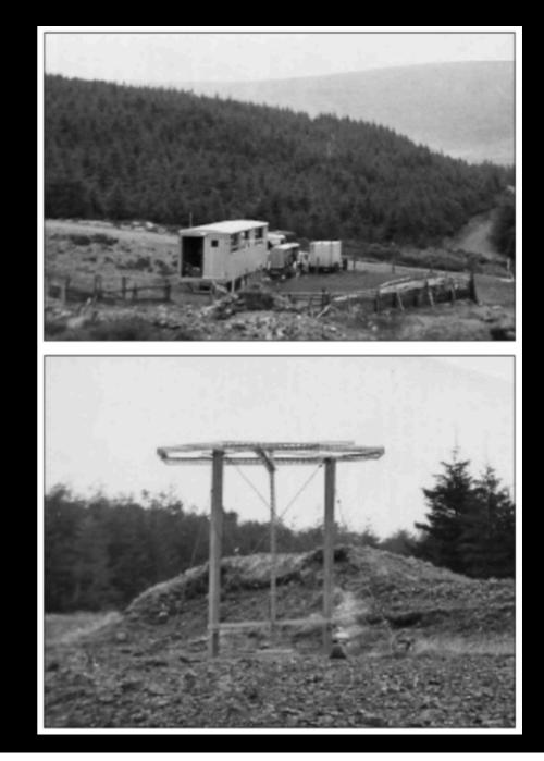
RADIO-ONLY EXPERIMENT IN UK (1969) WITH FOUR CONICAL ANTENNAS OPERATING BETWEEN 30 AND 60 MHZ, TRIGGERING AN OSCILLOSCOPE AND RECORDING CAMERA UPON COINCIDENCES BETWEEN PULSES FROM THE ANTENNAS.
