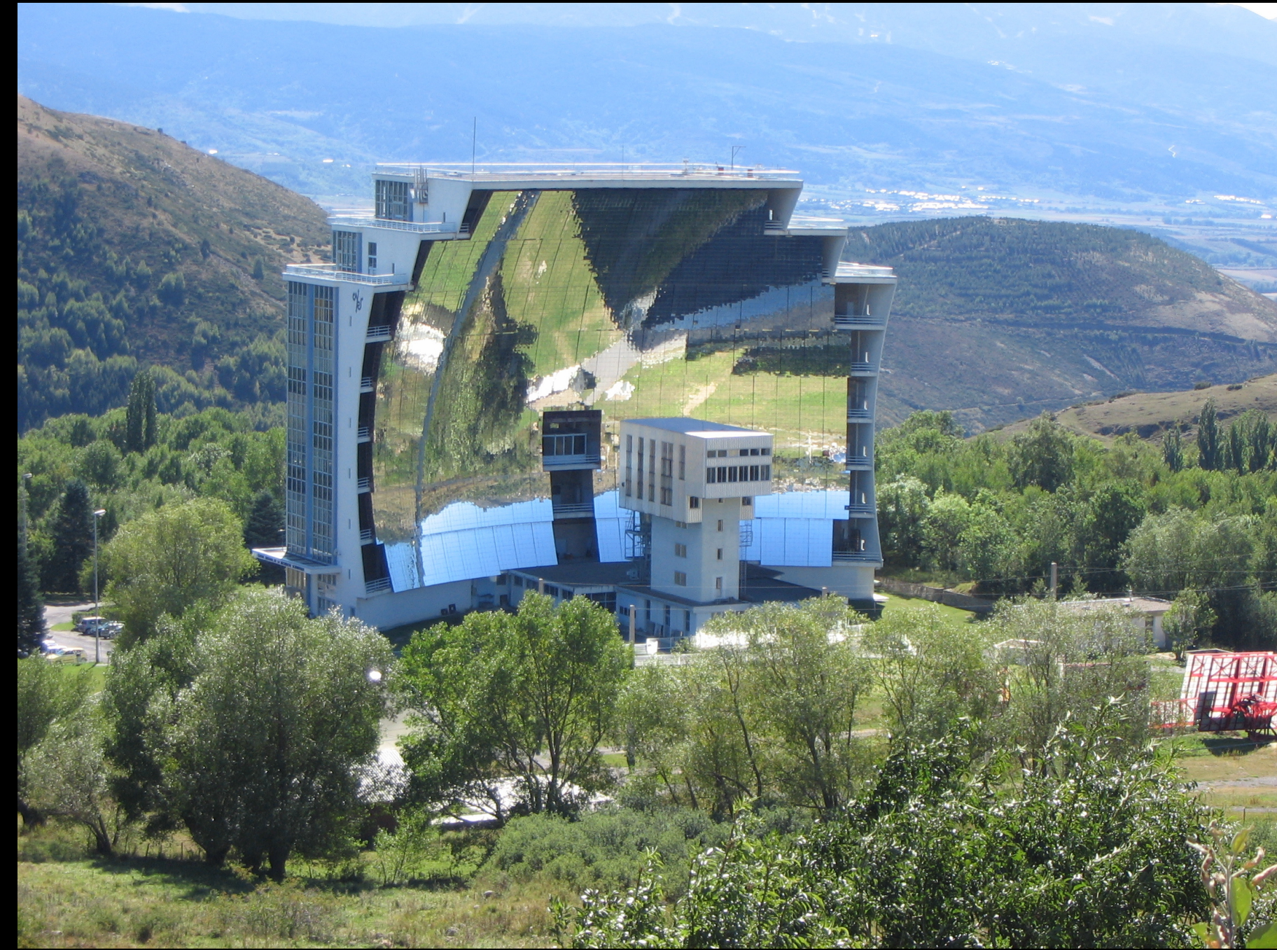
Odeillo facility (Pyrénées)
