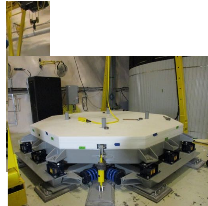
Seismic platform installation
