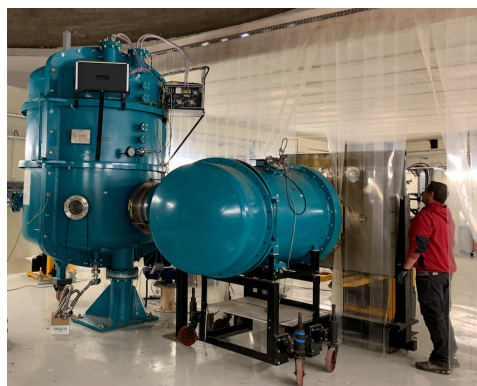
Fig. 5: Installation of the PERLE electron gun at IJCLab (Orsay, January 23).
