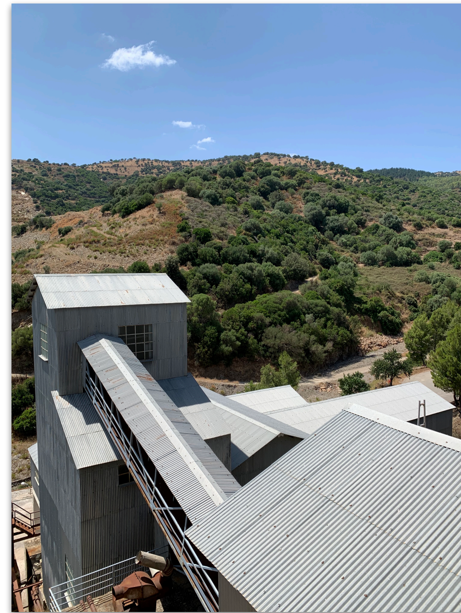
Former mineral processing unit
